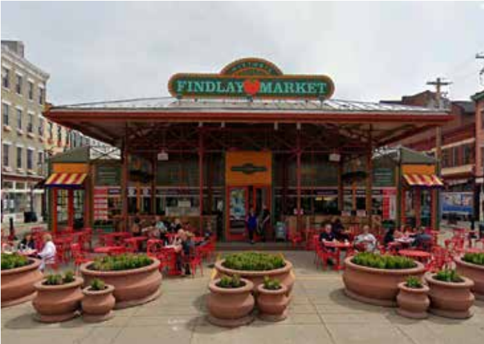
Retail Farmers Market: Findlay Market has helped catalyze mixed-use development in Cincinnati, OH
