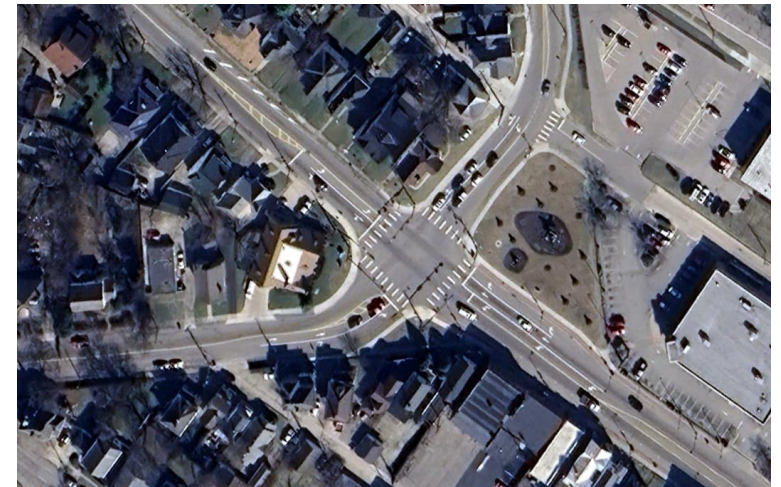
Figure 25: Main & Eaton Intersection AFTER Improvements
