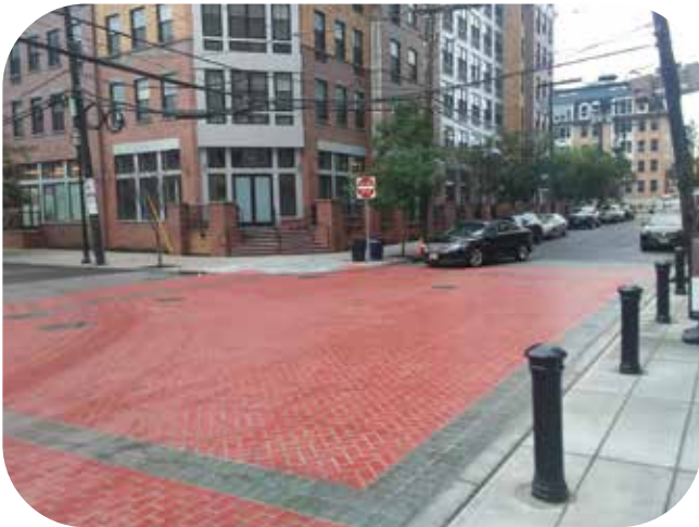
Brick Paved Intersection
