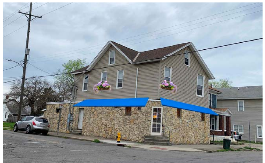
Rendering of the Potential Implementation of the Façade Improvement Program Along East Avenue
