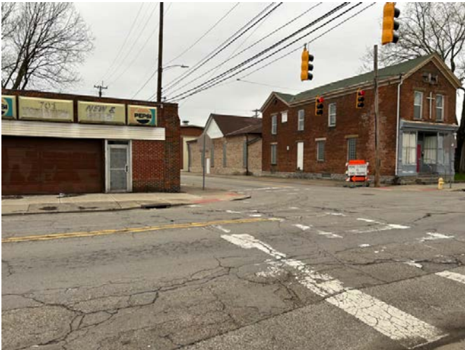
The Buildings on the West Side of the Intersection of East Avenue and Hanover
