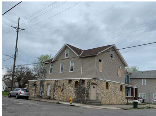
Current Building Condition
