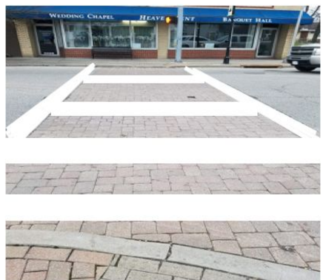
Recommended painted stripes on crosswalk to better alert drivers of pedestrian activity
