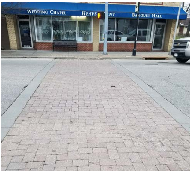
Existing conditions at Belle Avenue and Pleasant Avenue
